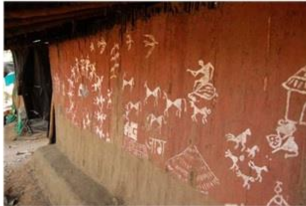
Photo 5: Bamboo purlins and mud plaster.
