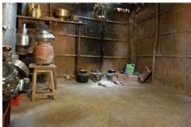
Photo 6: Thin bamboo walls and mud floor.
