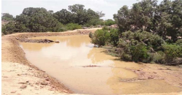
**Fig. 6 Rainwater harvested in a semi-circular bund**
