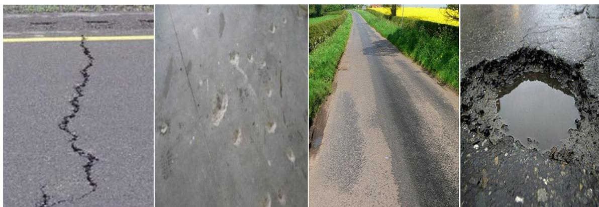
Fig : Example defects cracking, pop-outs, wear and polishing and potholes
