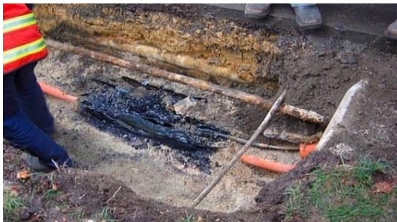
Figure 1: Example of underground cable fault.
