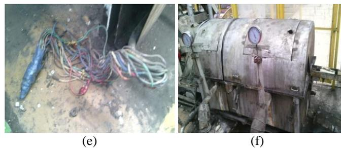
Figure 4.3(e, f): Poor maintenance of wiring and alkaline tank. As the alkaline tank is not properly maintained there is chance of tank to get bust up.
