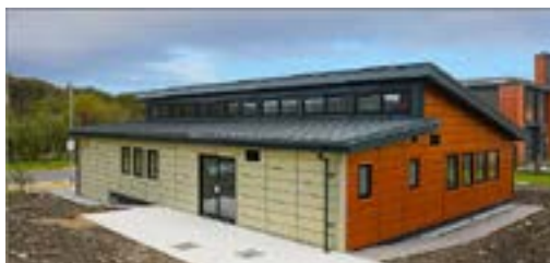
Figure: Active classroom based on Swansea University Bay Campus in United Kingdom with new generation of Colorcoat Prisma® Element (Seren Black, Seren Gold and Seren Copper)
