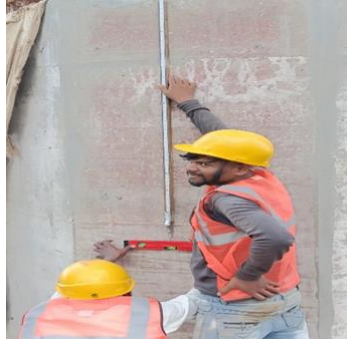
Figure 2. Checking the elevation.
