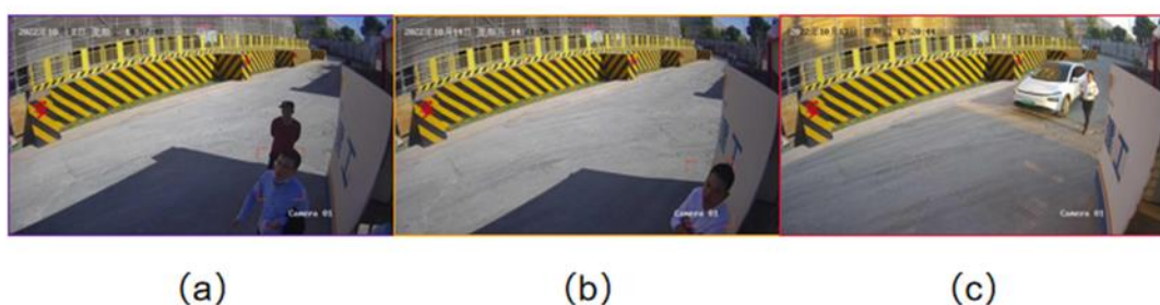
Figure 6. Three images reported on a construction site.
