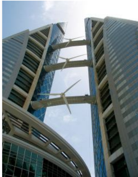
Fig. 1 wind turbine system integrated with tower building
