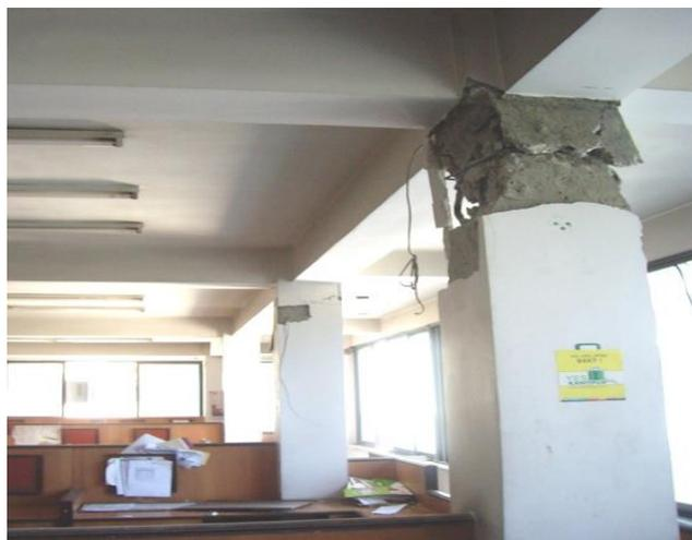
**Fig. 2.** Heavy damage to the top of the reinforced concrete columns at the level of the 2nd floor of Building No. 2 Media-TV center "Kantapur" in Kathmandu in the Republic of Nepal in the catastrophic earthquake in April 2015, Building No.1 was slightly damaged.
