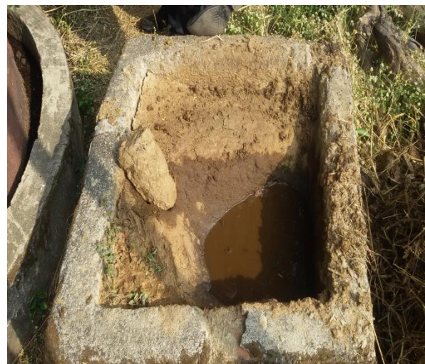
Fig. 1 Present physical status of biogas plans due to faulty construction and poor workmanship
