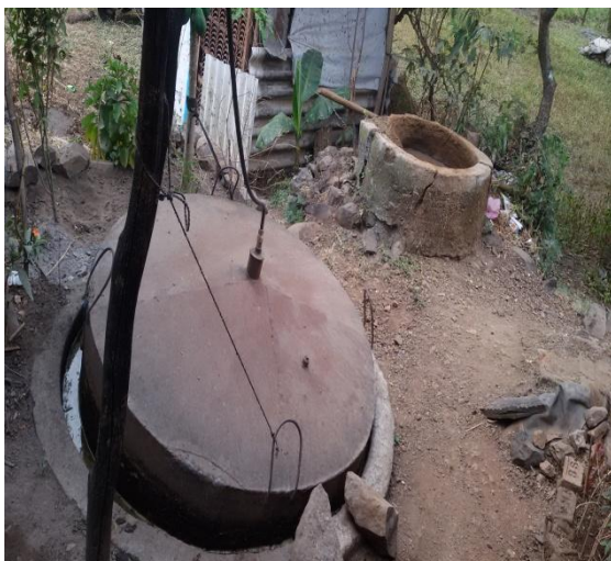
Fig. 1 Present physical status of biogas plans due to faulty construction and poor workmanship
