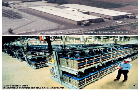
Fig9: Battery energy storage system
