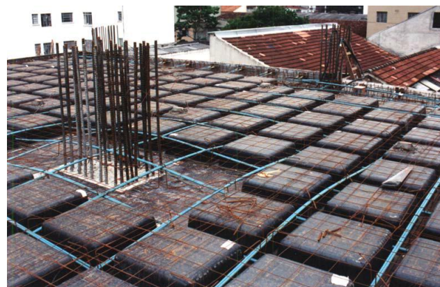
(b) Post-Tension Waffle Slab
