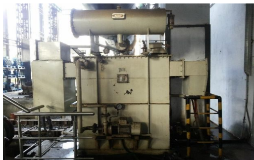
Fig.1: Front view of 2500KVA HT Transformer
