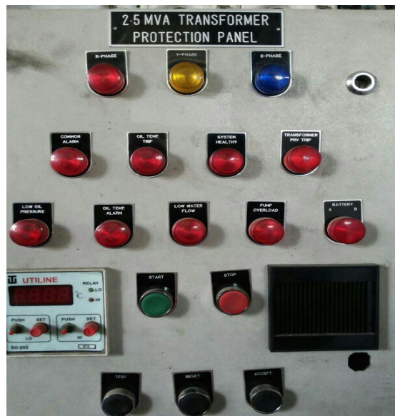
Fig. 3: Front view of Digital control panel showing the Audio-visual indications.
