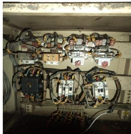
Fig.12-b Contactors used for speed control
