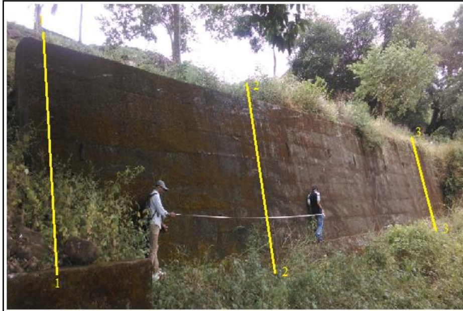
Plate 1 Existing Retaining wall at Dewarwadi
