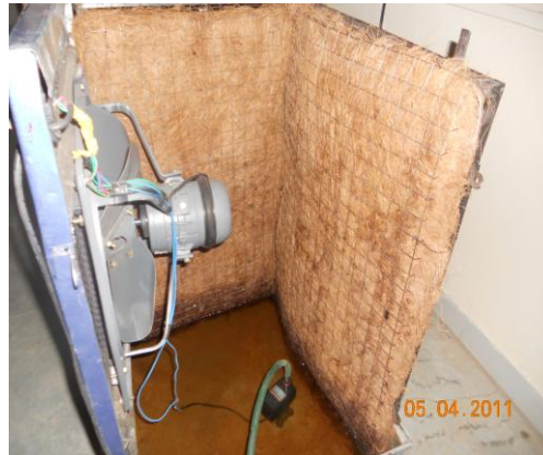
Fig. 5 Test rig of Evaporative cooler
