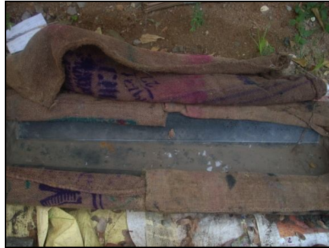
Fig. (9) Curing of panels
