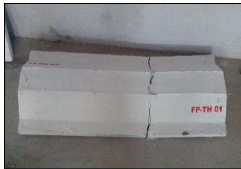
Fig. (13) Crack pattern (FP-TH 01)
