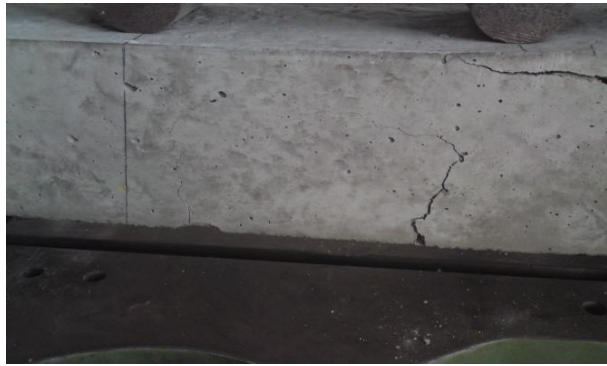
Figure 3. Crack propagation while loading
