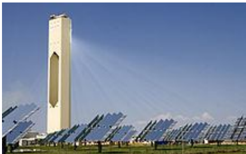
Figure 1. Concentrated Solar Power System
