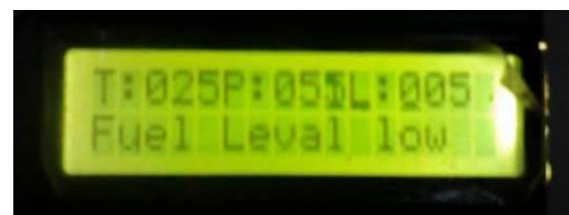
Fig 9. Fuel level low alarm
